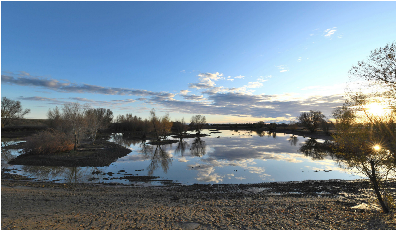
Woodland Regional Park wetlands construction site. Photo Credit: Lars Anderson
